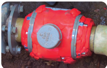
Split Sleeve Repair Photos
